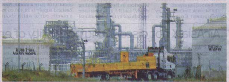
A view of the Refinery and Petrochemical Integrated Development (Rapid) oil refinery at Pengerang Integrated Petroleum Complex. Photo: Reuters
